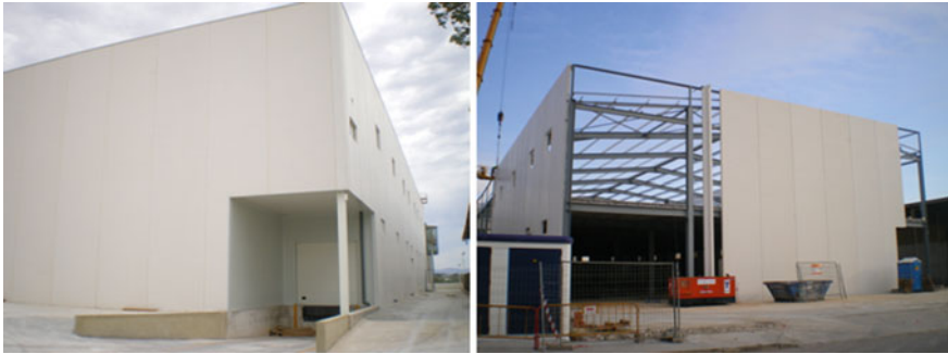
Fig. 4 Industrial plant images Source Elaborated by the authors
