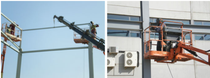
Fig. 5 Structure Works Source Elaborated by the authors
